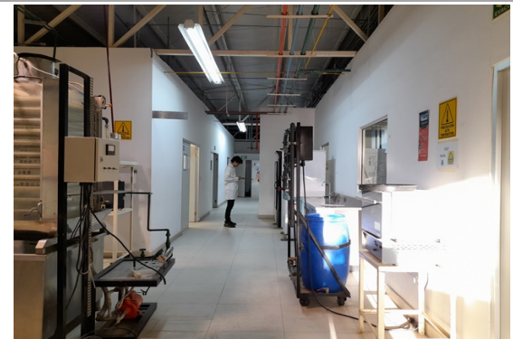
F5: Pasillo interior
