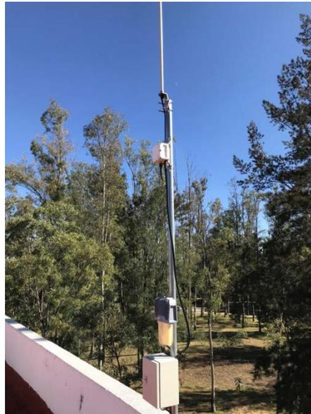
Figura 7. Antena PROCOM CXL900-3LW
